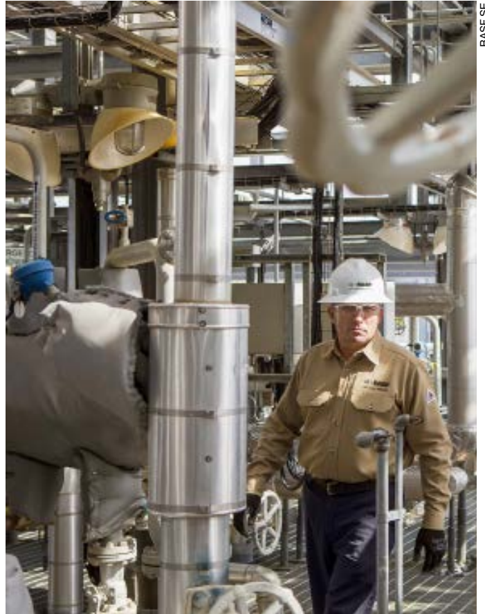
BASF, Wyandotte, Michigan, plant commissioning by CH2M Hill
