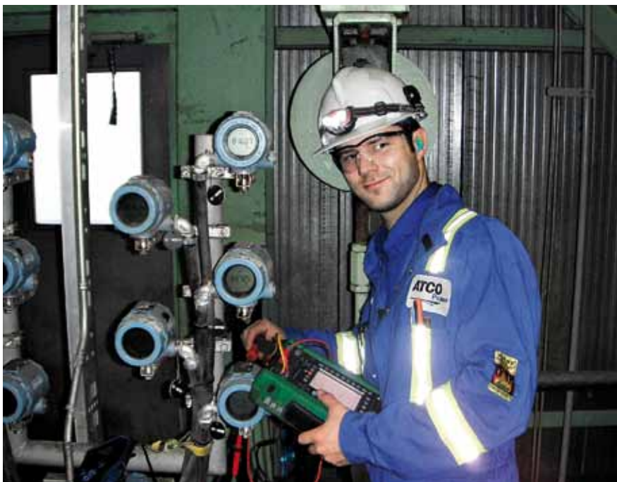
Shane Haugen calibrating a transmitter with MC5.
